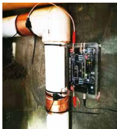
Vulcan S10安装在总出水管道上
