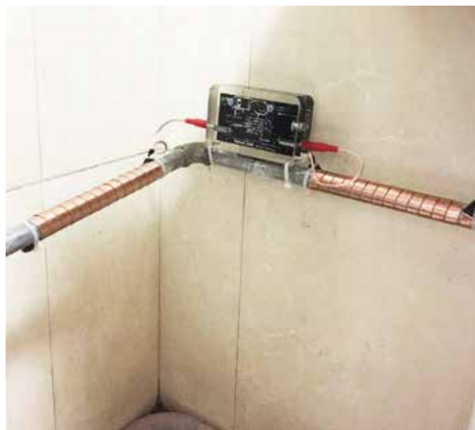
Vulcan 3000安装在学生宿舍里较小的管道
